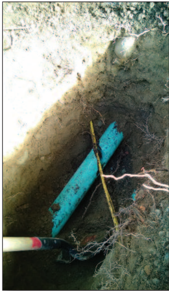
Gas line through sewer lateral
