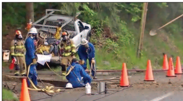
Blowing 6 inch IP repair, shovel launched by gas pressure
