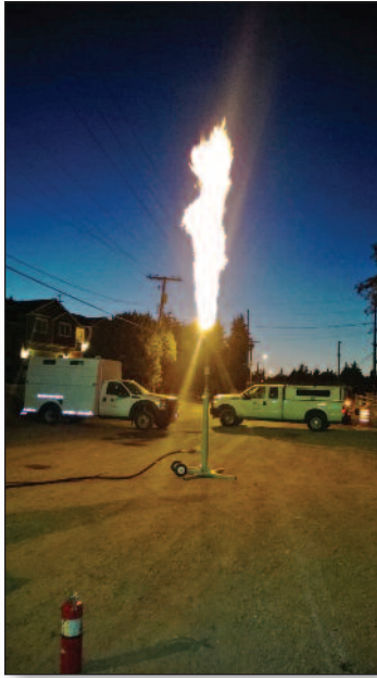
High pressure gas flare off
