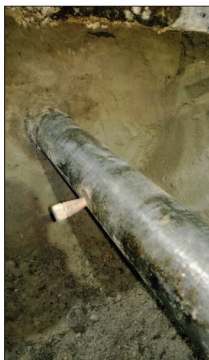
Boiler plug pounded in to stop a leak
