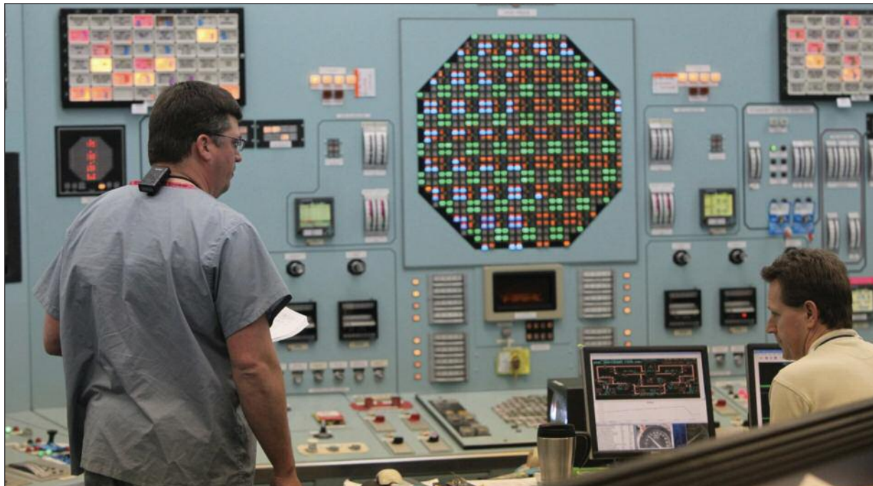
Workers inside the control room of the Columbia Generating station nuclear plant that has a simulation of the fuel core on the wall. (Steve Ringman/The Seattle Times)
