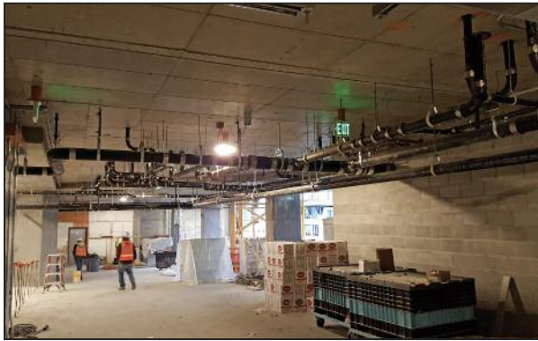
Holmberg Company Project: Tower 12 - Cast Iron Waste System
