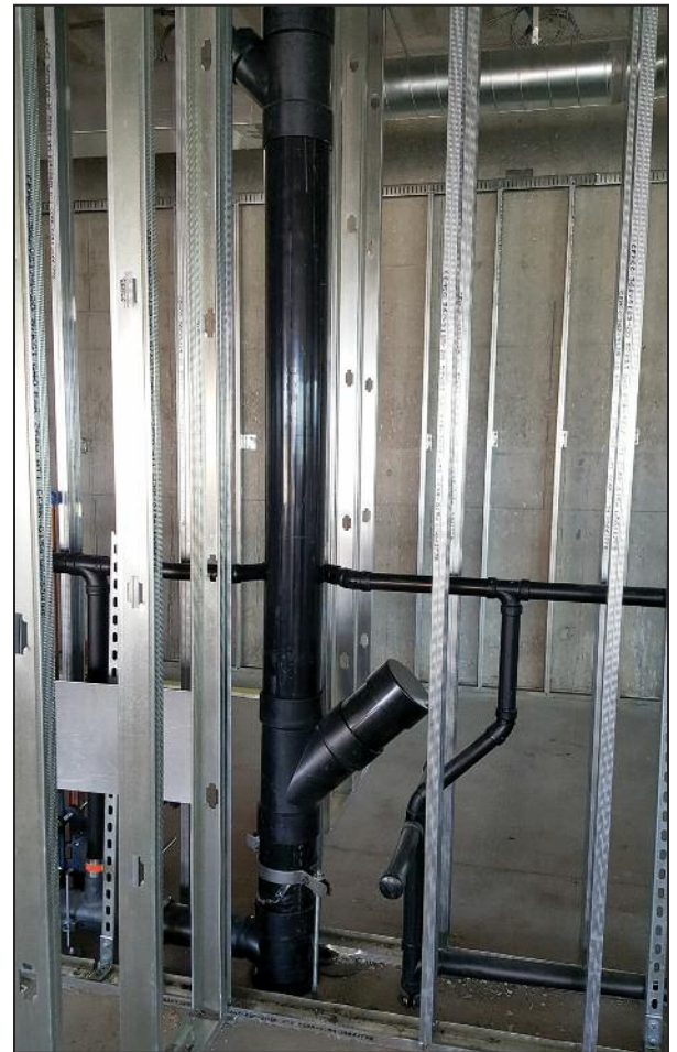
425 Centre in Bellevue ABS Waste Stack - Things have changed!
