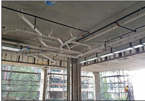
Hawk Mechanical Project: PVC Waste Piping - Marriott Hotel Bellevue
