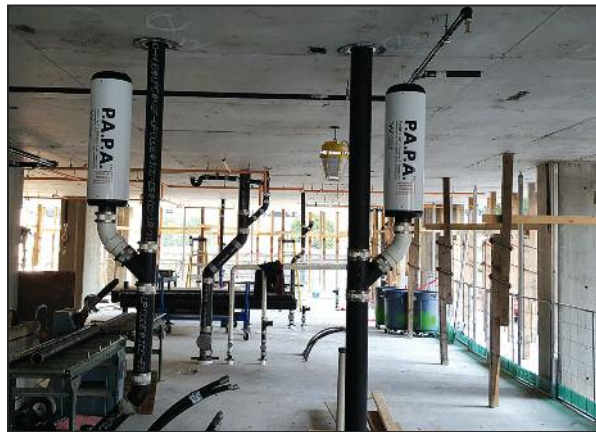
Positive Air Pressure Attenuator. These devices eliminate Yolk Vent Piping – at Tilt 49, a Hermanson Project
