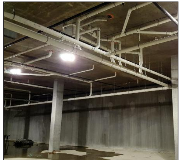
Drainage Piping – Ocean Park Mechanical Job on Westlake Ave.
