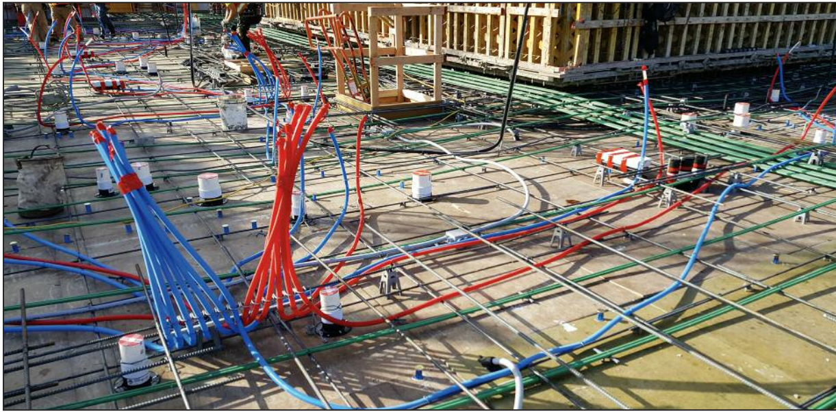
Inserts, Piping & Sleeves on the 34th floor of the Kinetics Project- Holmberg Company
