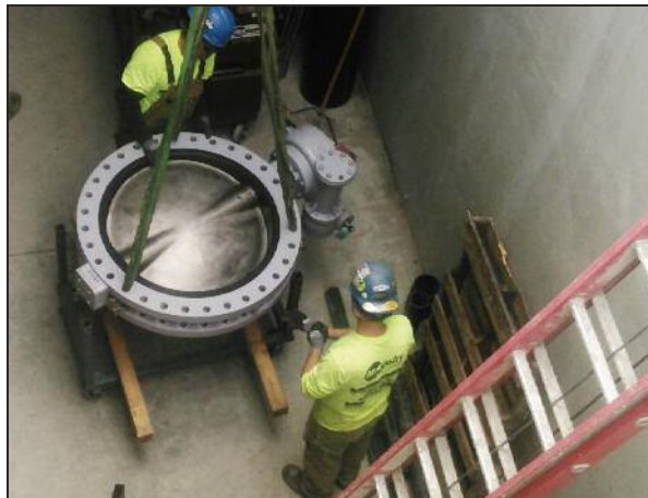
Brothers Scott Durance and Robert Rivera landing a 36" butterfly valve at UW CUP
