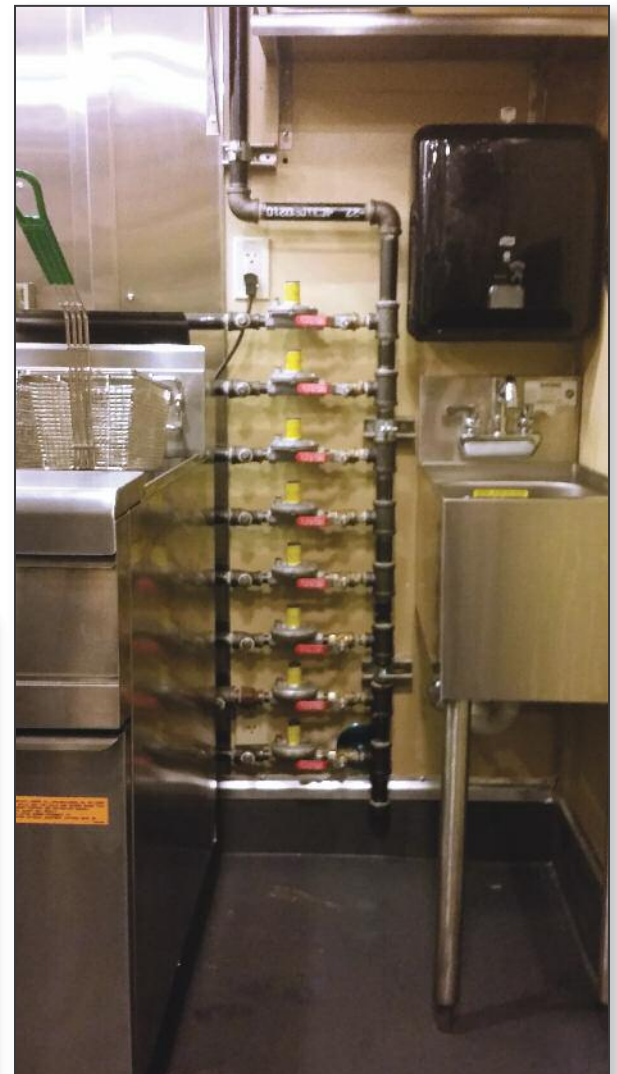
Gas Pipe Header at McMenamins-Bothell one of three Full Size Kitchen
