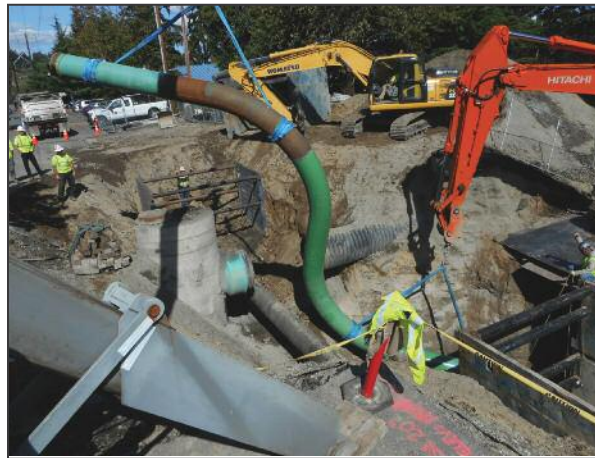
Brothers Cody Hinman & Curtis Ary setting their Fab for Hydro-test & Prep Tie-ins
