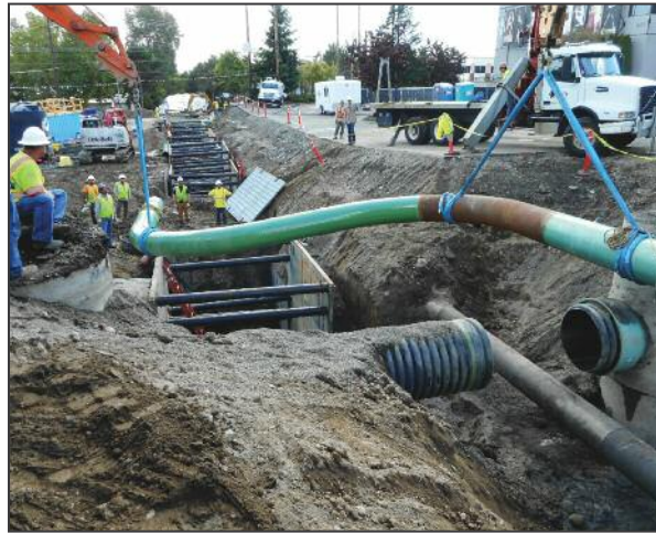
Brothers Cody Hinman & Curtis Ary setting their Fab for Hydro-test & Prep Tie-ins
