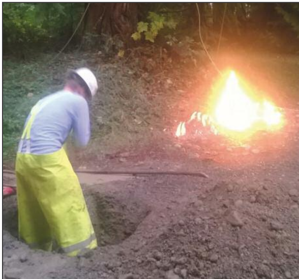
Local 32 Fitter working to shut down 2" main gas line damaged by an arc burn.
