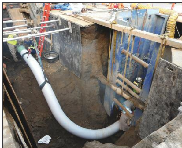
UA Members doing Final Tie-ins for BP Olympic Line Shut down
