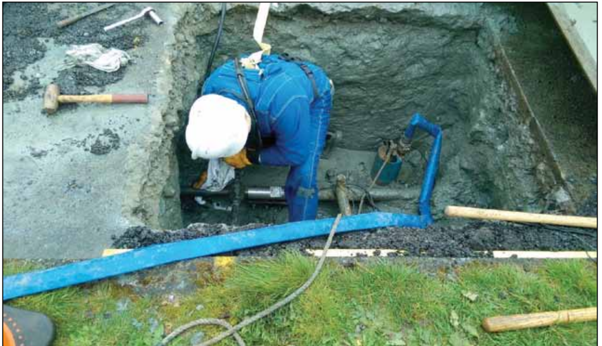
UA fitter in breathing air installing a leak clamp on blowing P.E. gas main.
