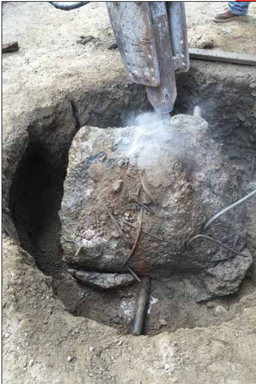
Crew stands by while concrete is broken around steel gas main.
