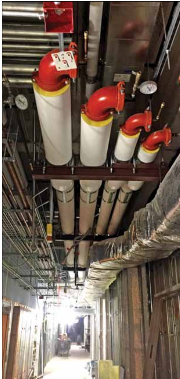
Prefabricated pipe rack installed at Covington Multi-Care for UMC
