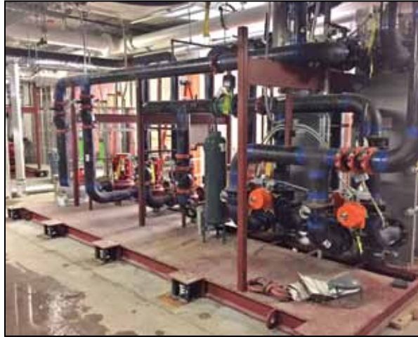
Prefabricated skid installed at 400 Dexter for PSF Mechanical
