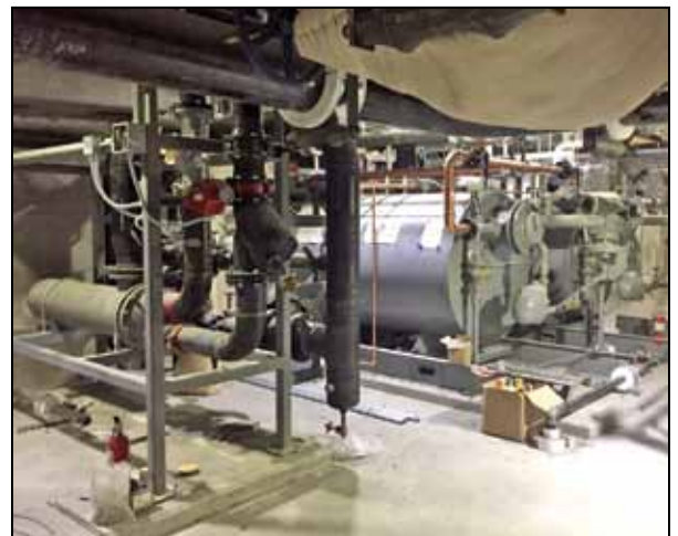
Boilers and heat exchangers in mechanical space at UW ARF for MacMiller
