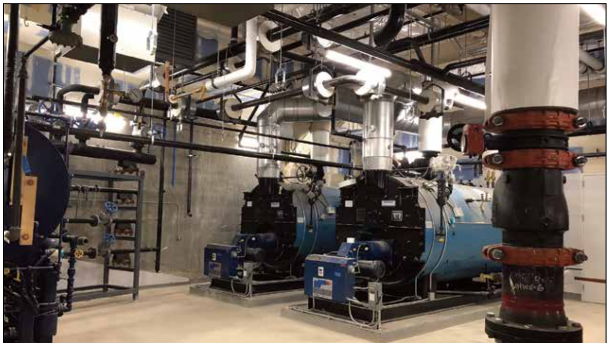
Steam boilers installed at 8th & Howell for MacMiller.
