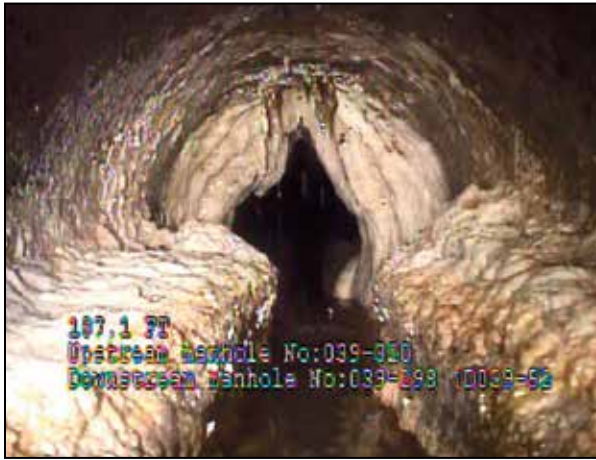
This concrete sanitary waste line has to be jetted and scoured every 6 months to prevent blockage!!!
