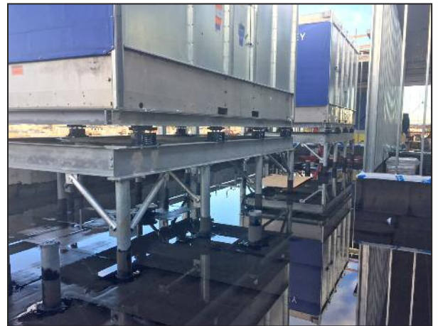
McKinstry cooling tower—Cooling Tower and prefabricated supports built in McKinstry's shop installed on site at UW Medicine 3.2."
