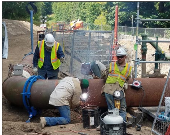
Snelson Crew welding in a double stopple bypass to install new 30" Block Valve
