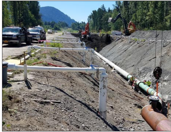
Abercrombie Welders laying 30" heavy wall in 24' deep ditch
