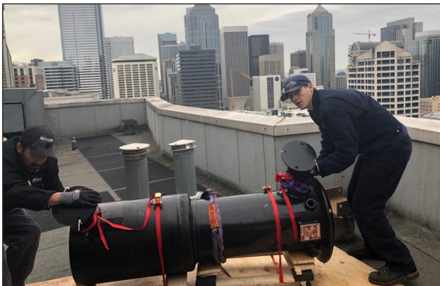
McKinstry replaced a 880# boiler heat exchanger on a rooftop downtown.
