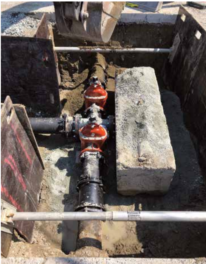
Water main extension installed by Local 32 members working at SPU.
