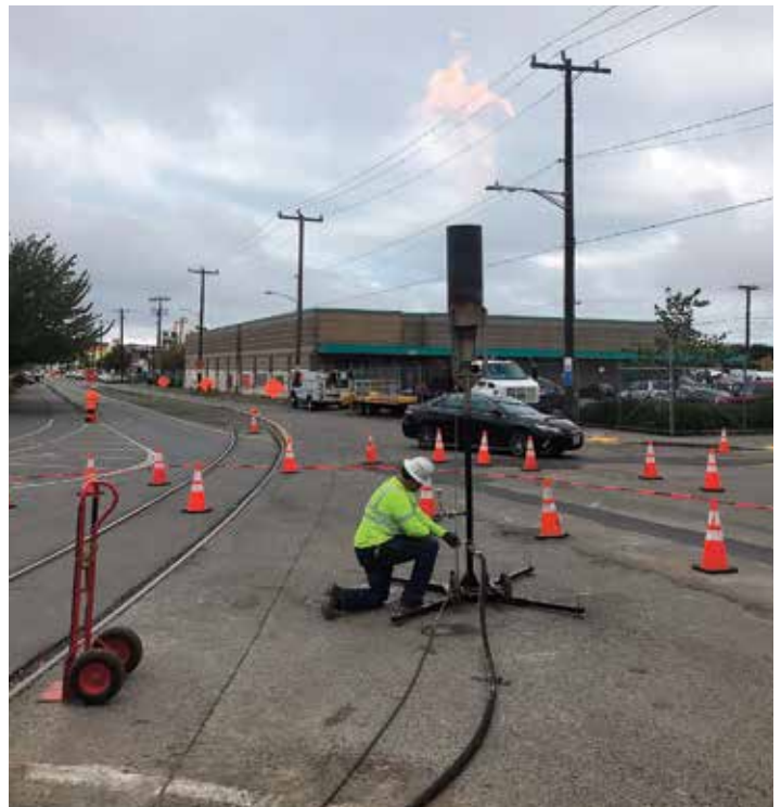
Natural gas high pressure flare.
