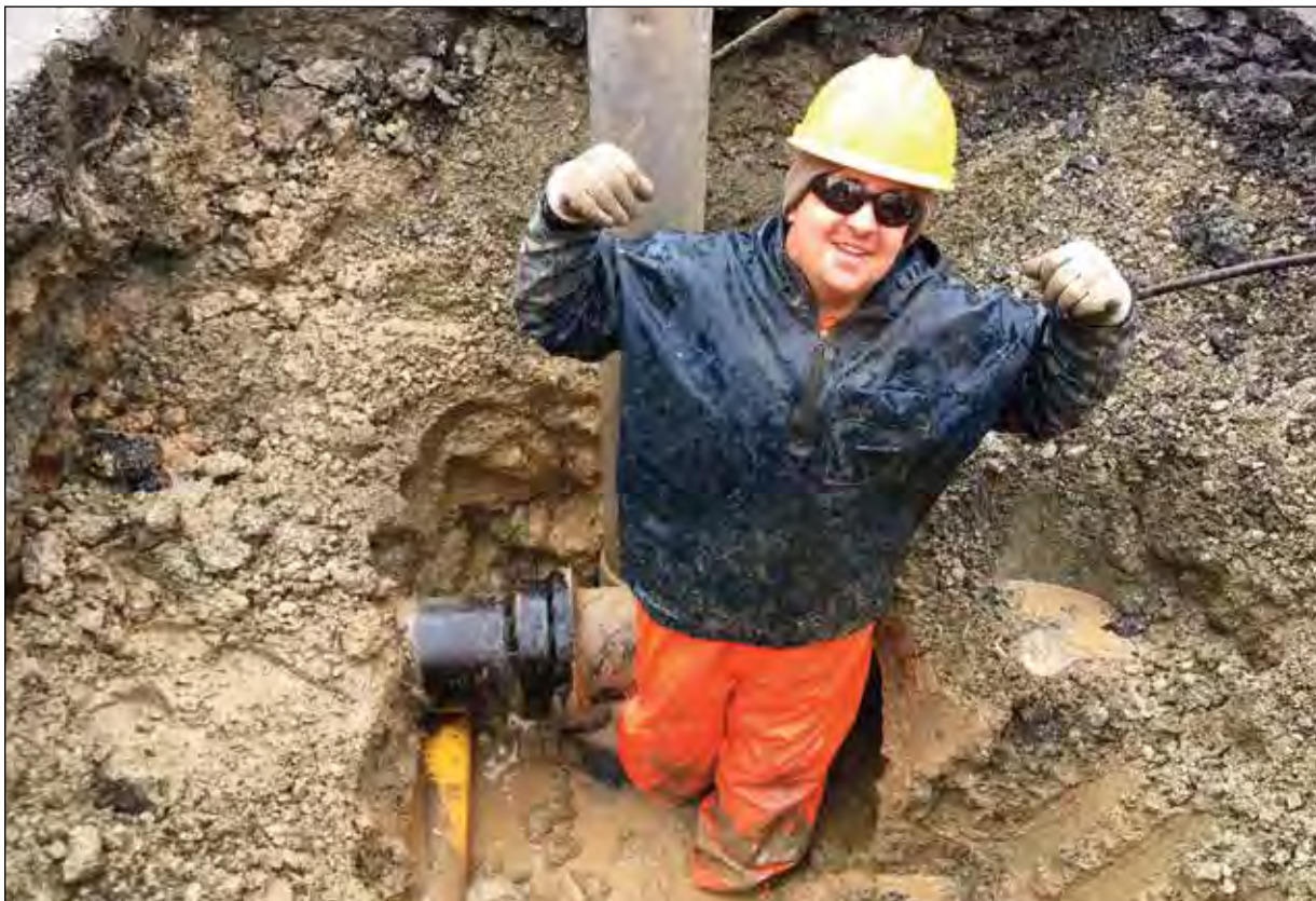
Local 32 Member Eric Ankerfelt working an 8" cast iron bell leak.
