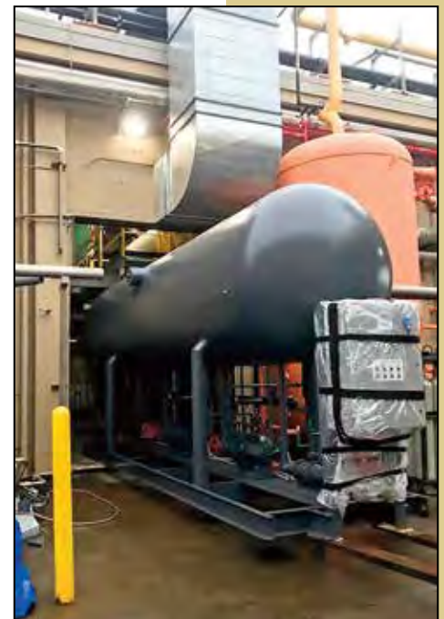
Permacold moving a Low Pressure Receiver into the Safeway ammonia plant in Bellevue.
