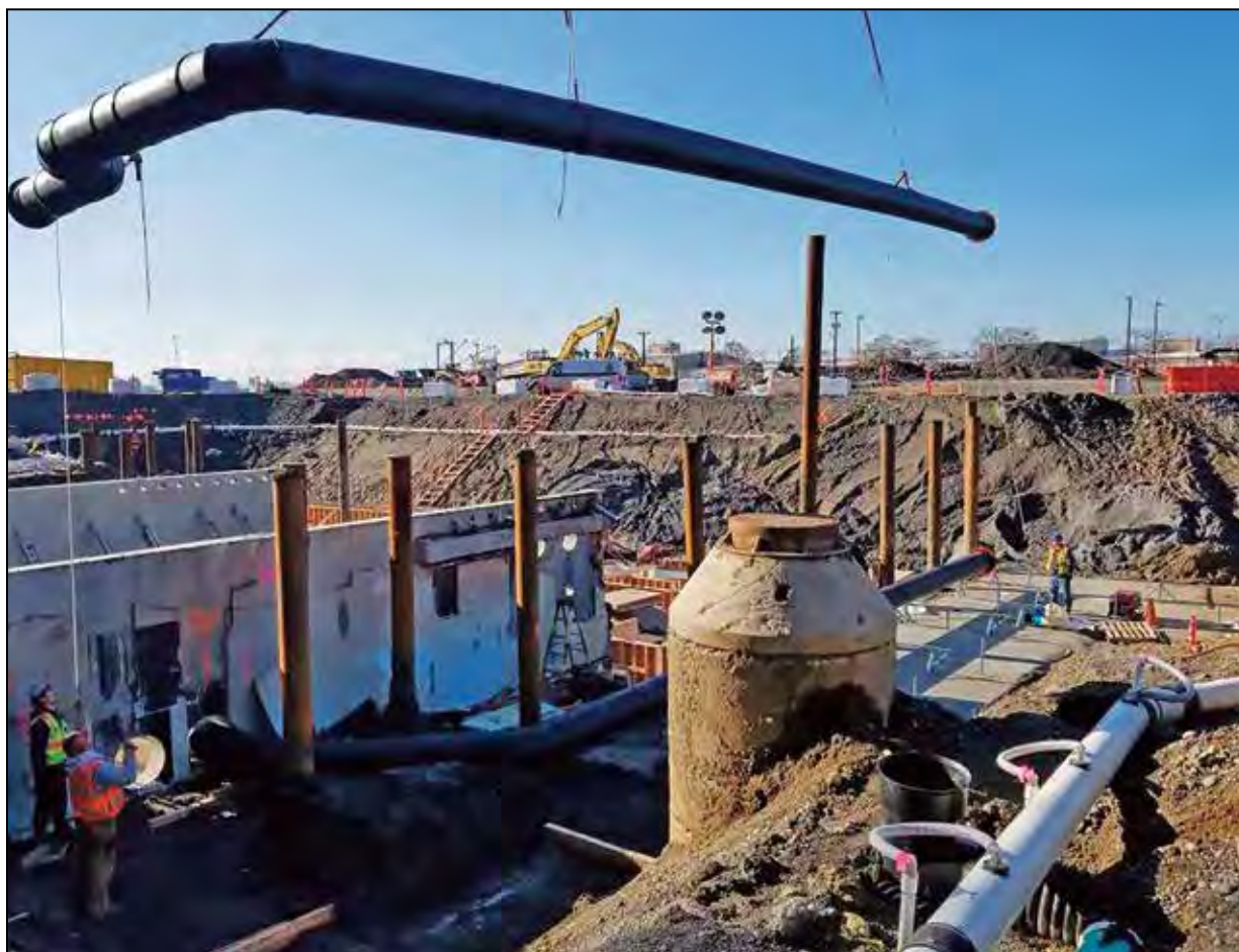
Local 32 installing 30" HDPE at the Expedia project
