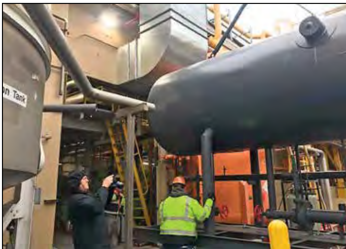
Permacold moving a Low Pressure Receiver into the Safeway ammonia plant in Bellevue.
