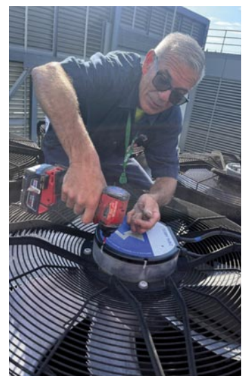
Long time mechanic Terry Gangwish of McKinstry working on a fan motor replacement
