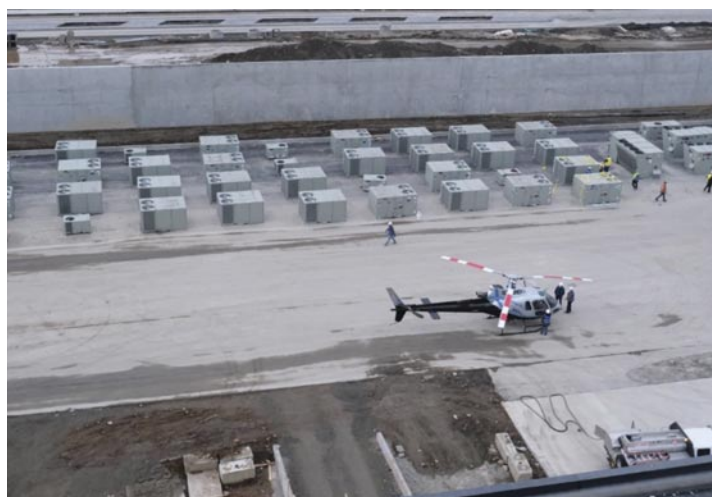
Joe Sparks of MacMiller and the crew landing units on a rooftop with a helicopter. They set 60 units in 6 hours.
