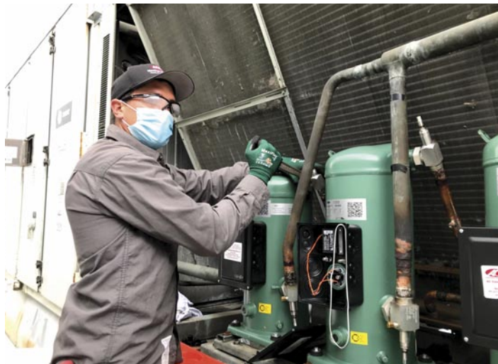
Brendon Thorstad and Zack Burgy changing out a bank of compressors on RTU
