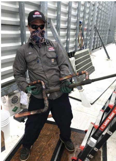
Brendon Thorstad and Zack Burgy changing out a bank of compressors on RTU
