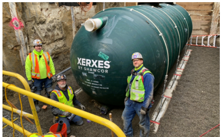
Rainwater Catchment Tank (left to right) – Steve Johnson, Joel Stillings, and Paul Deines securing a 9,000 gallon rainwater catchment tank.
