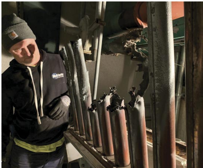
Greg Koch with a mangled RBI burner on a late-night emergency boiler repair at a Bellevue hotel
